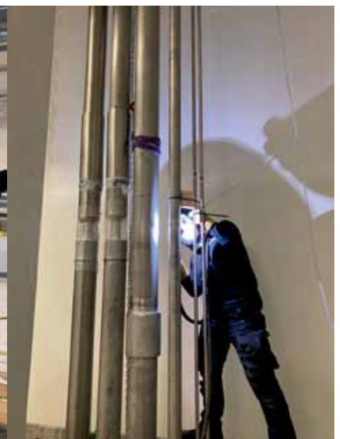
Demaco's mechanics performing installation works at ESS site. Welding of a vacuum insulated transfer line site connection to the left and welding of uninsulated piping to the right.
