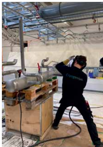
Demaco's mechanics performing installation works at ESS site. Welding of a vacuum insulated transfer line site connection to the left and welding of uninsulated piping to the right.
